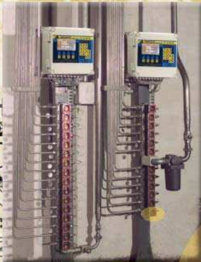
Typical Flow master assembly
