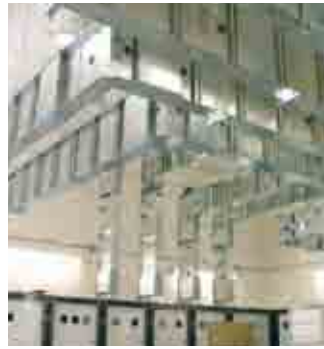
Switchboard-transformer connections
